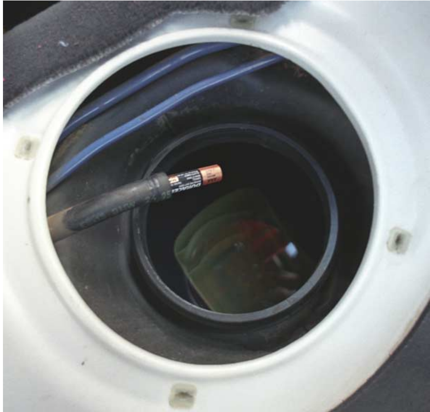
Figure 10: View Inside rhs Tank -- Reserve Sump
